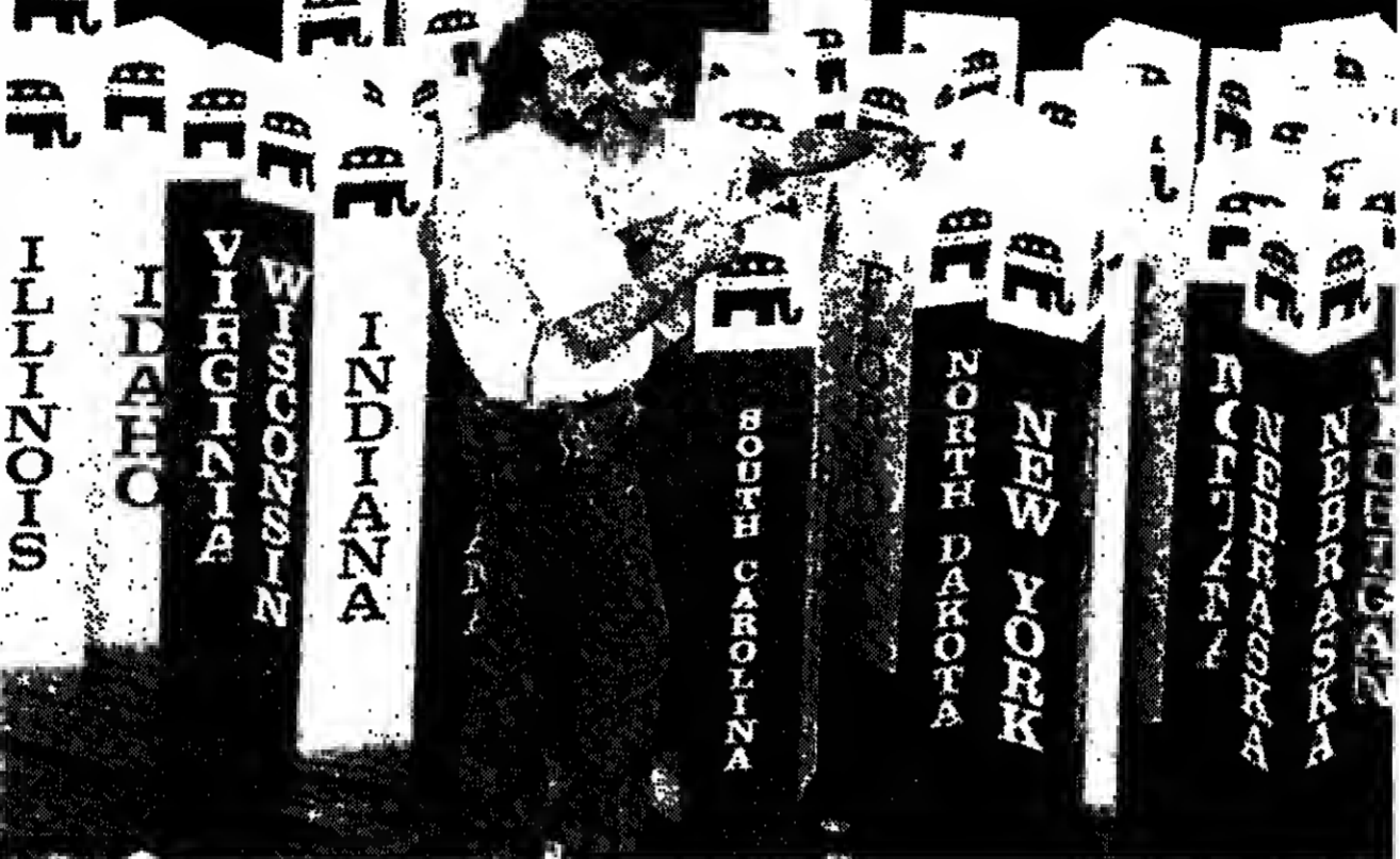
Workers at the site of the Republican National Convention in New Orleans sorting out signs for the state delegations.
